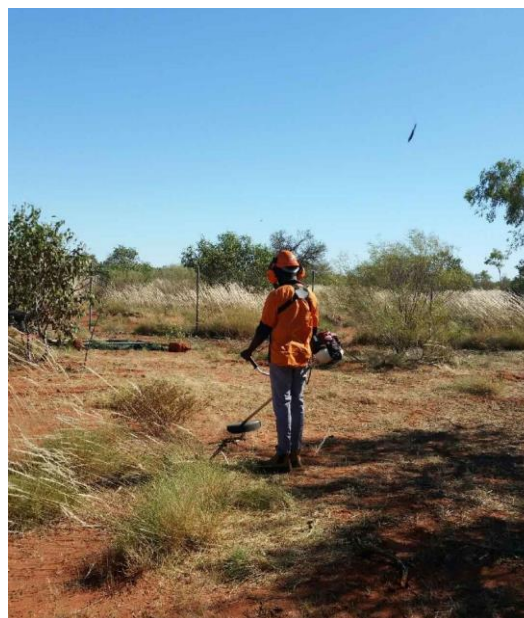
Clearing the Training Centre grounds
