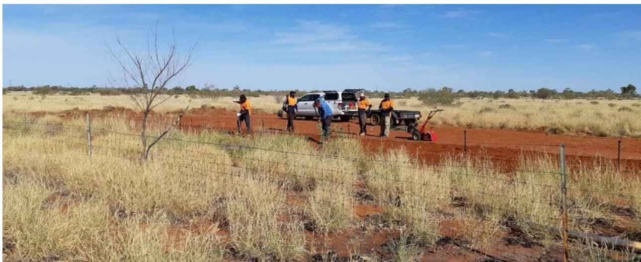
AHPL staff installing irrigation line at the farming area
