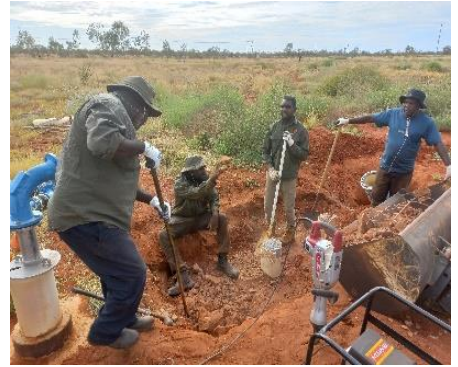
Installing the irrigation mains from the bore
