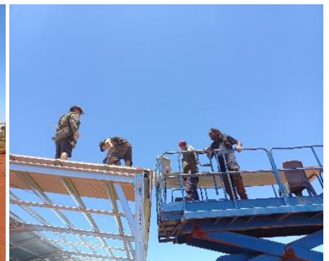
Building a shade structure for the classroom
