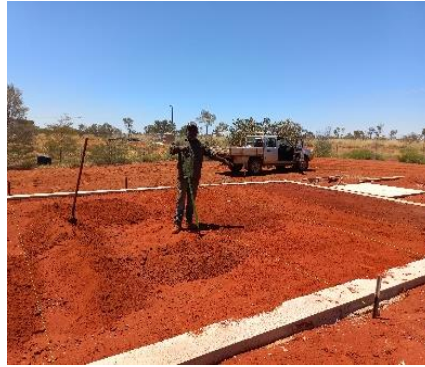
Establishing footings for the greenhouse
